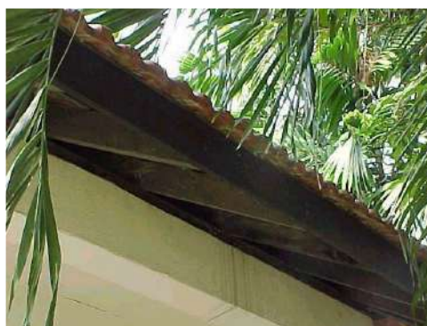
Fig.5.4 Removal of unserviceable roof gutters
